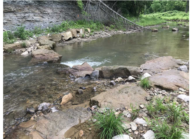
Photo: Cross-vane at East Fork Indian Creek
